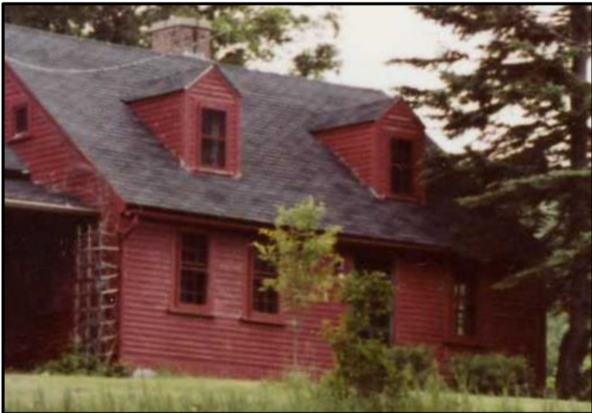
Compare West Fairlee home in 1981, seventy-two years later. Dormers were added in roof.
